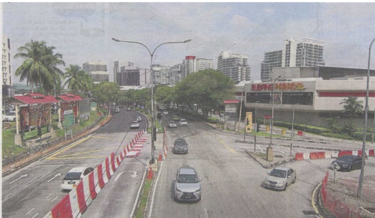
The roadworks are required to take place before any further development of the area can be carried out.
