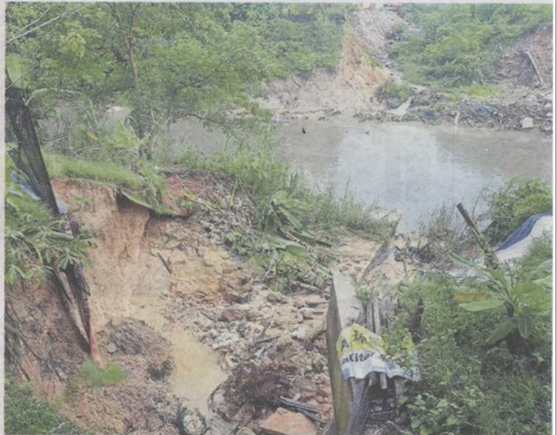
The riverbank near Jalan 1A/26D, where traces of the main drain outlet (concrete structure in foreground centre) can still be seen.
